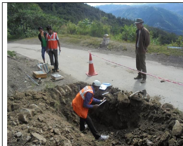
Measurement of pavement thickness at Km 59+000 LHS
